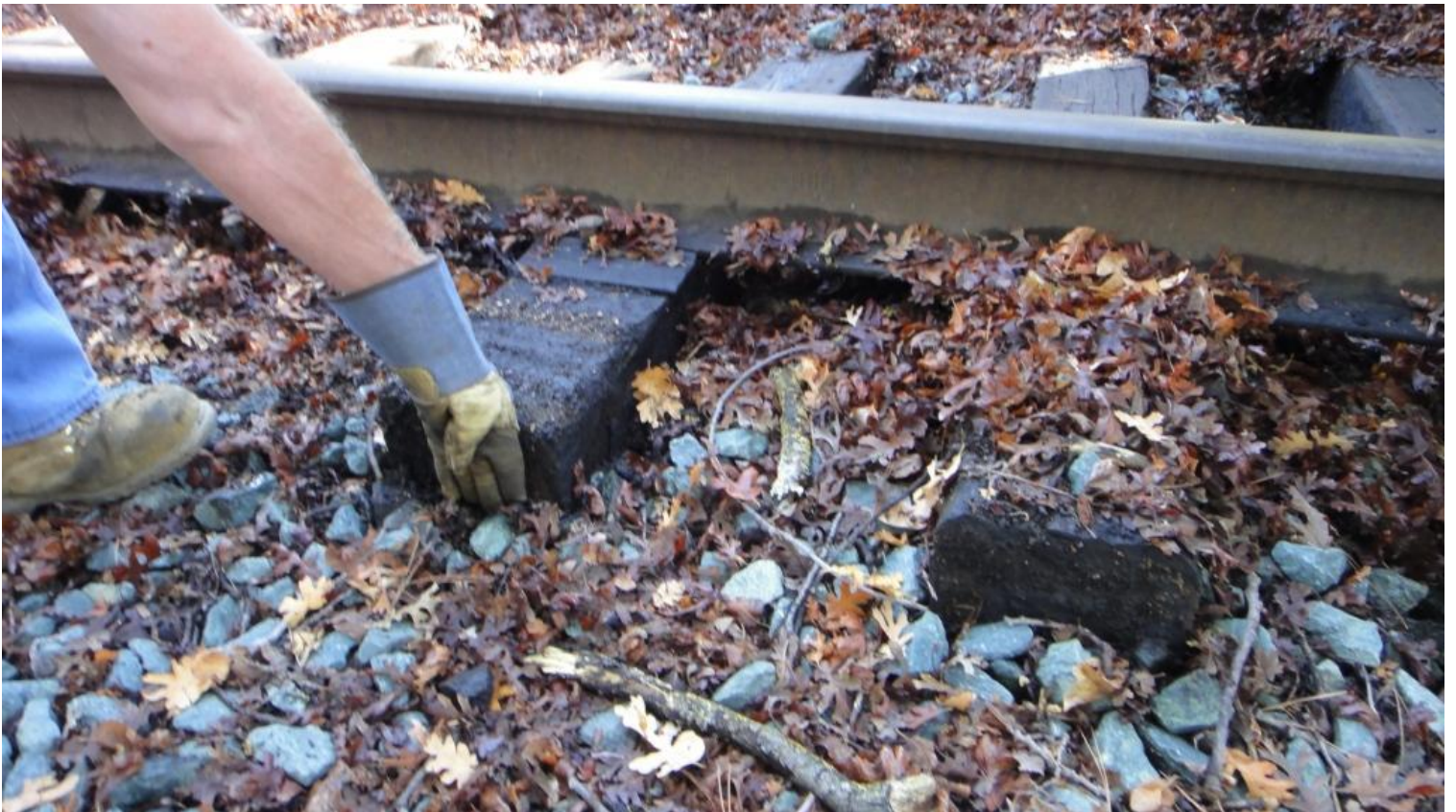
Clem demonstrates how high the J3K lifted the track – now if we only had some ballast...
