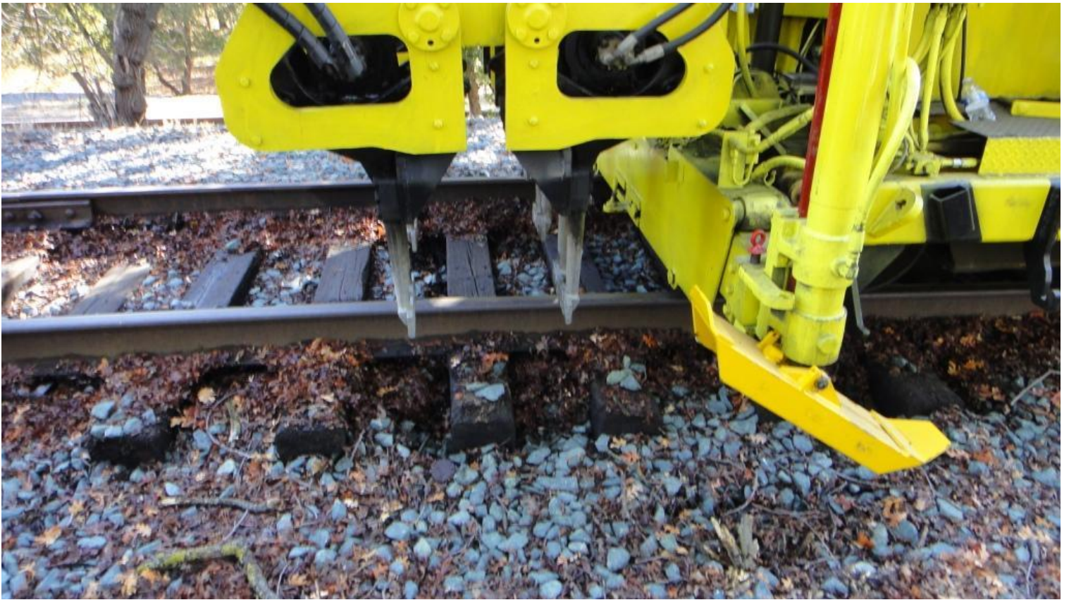
The track has been jacked
