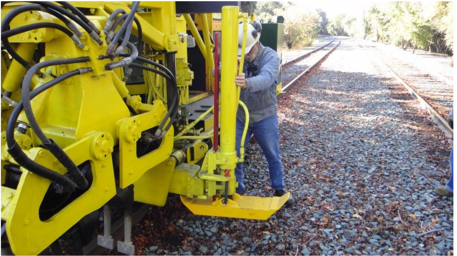
Alan bringing the lifting jack of the J3K into position
