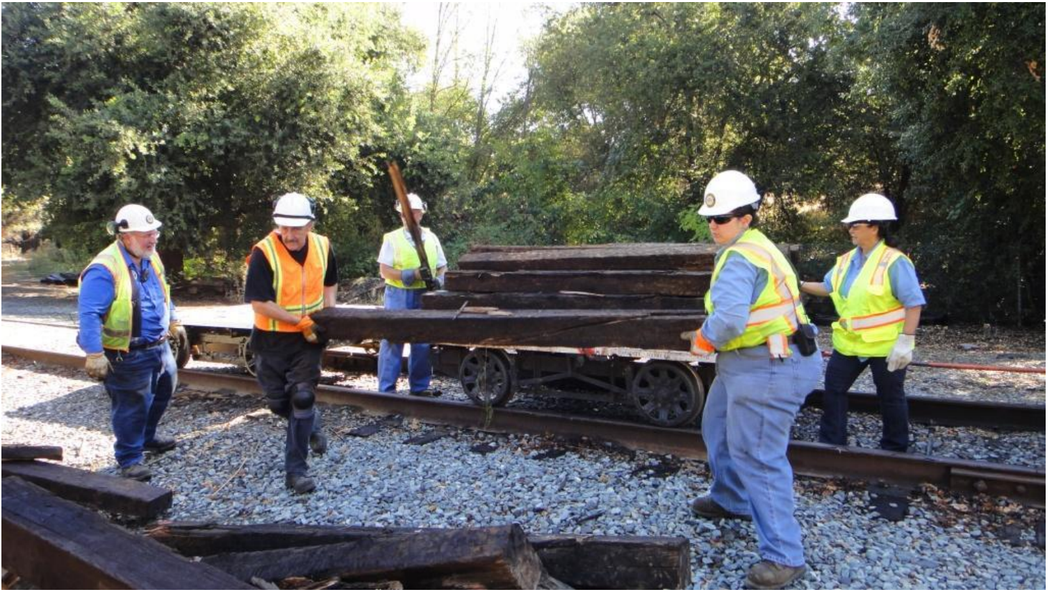
Meanwhile, down at Setzer, Frank, Fred, Clem, Heather, and Pam dispose of dead ties
