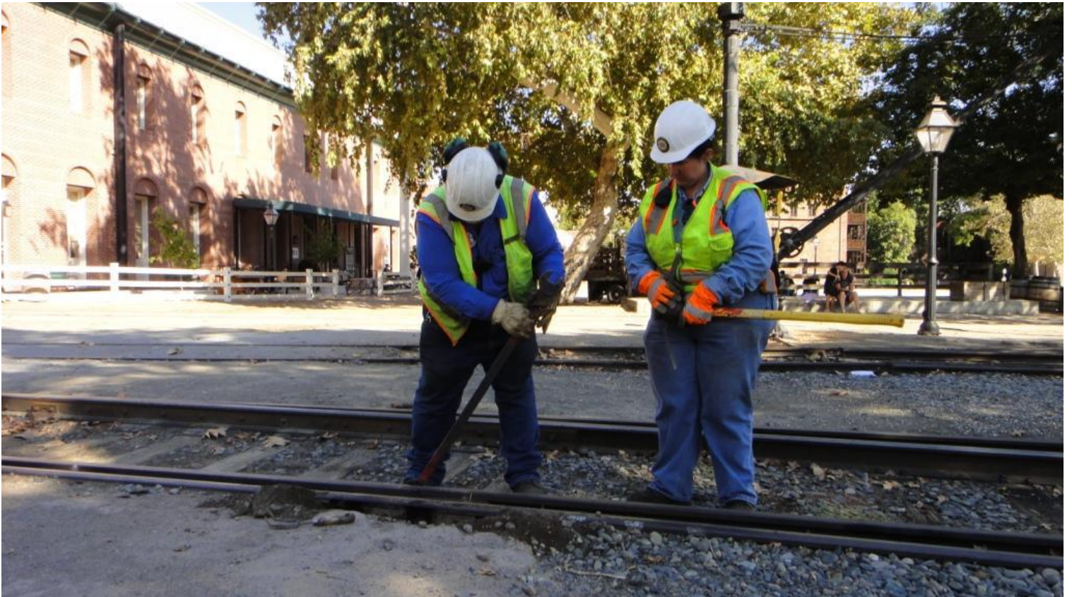
Frank and Heather secure a loose joint-bar near the stub switch
