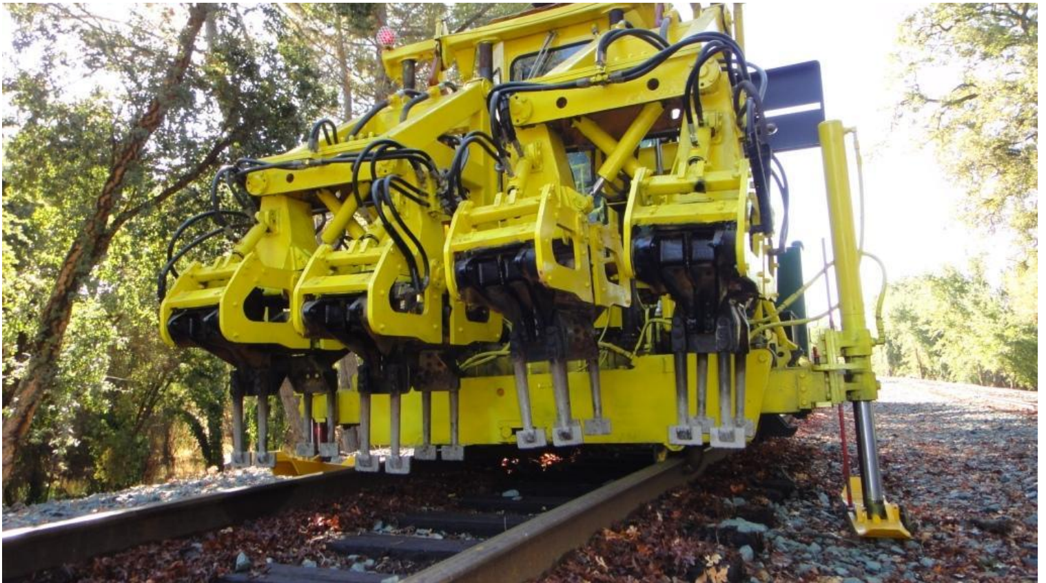
The rail-grabs are engaged as the jacks are deployed
